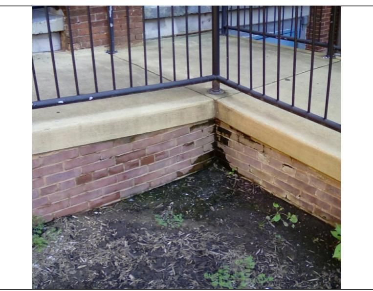
(5) Water damage due to drainage patterns
