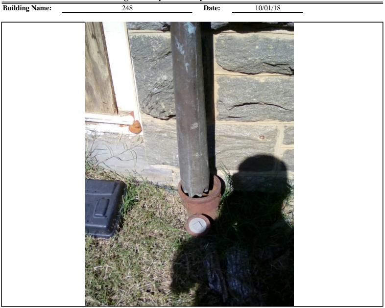
(10) Roof drain downspouts do not go far enough down into the underdrain pipe.
