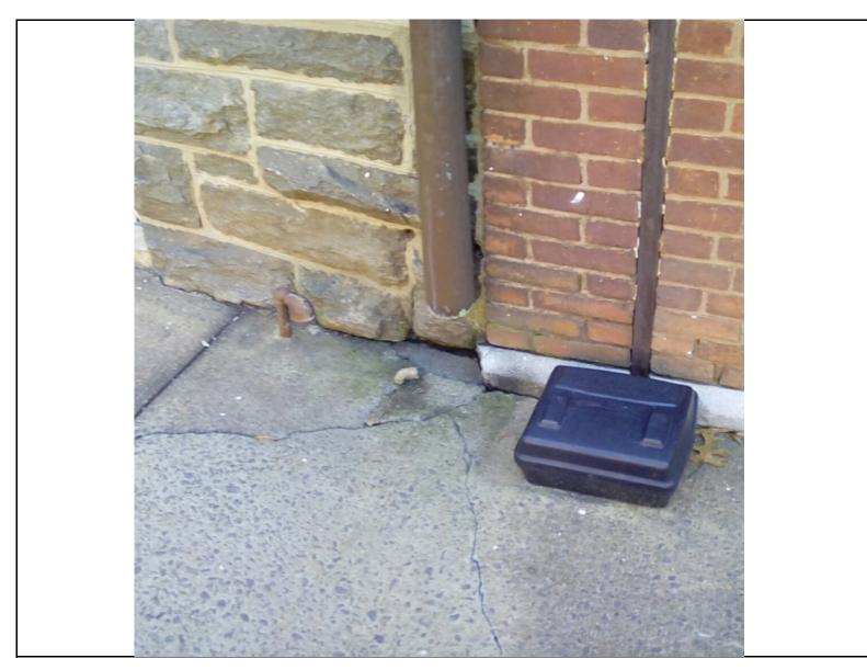
(7) Roof drain outfalls directly to sidewalk with no 45 degree connection.
